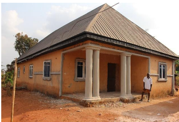
Mr Alexander Okhilua newly built 4 bed room bungalow house
